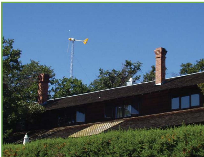
The 10 kW Bergey wind turbine provides about 30% of the farm and ranch's annual electricity needs.
